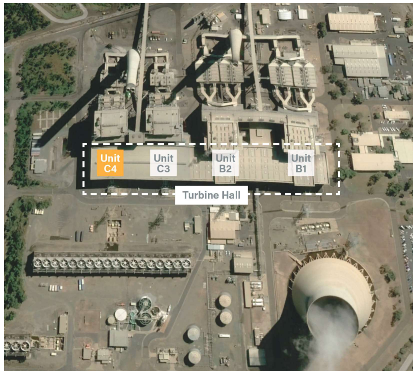
Figure 3 Site layout of Callide C and B power stations showing position of turbine generators
