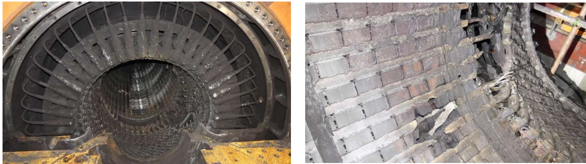
(a) Generator stator internal condition
