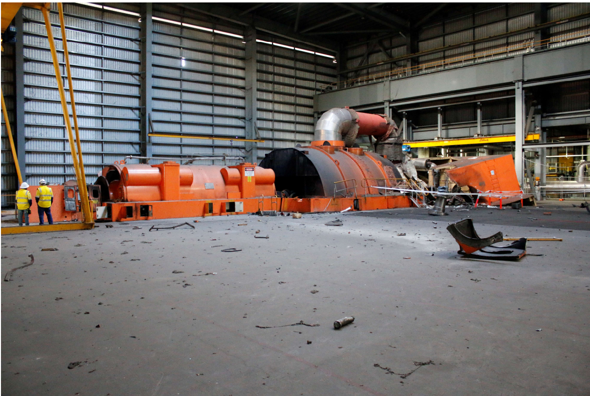
Figure 35 Post-incident damage to Unit C4
