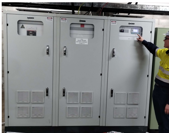
Figure 62 Unit C4 battery charger
