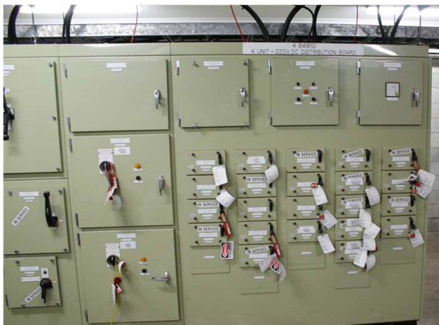
Figure 67 Unit C4 DC distribution switchboard
